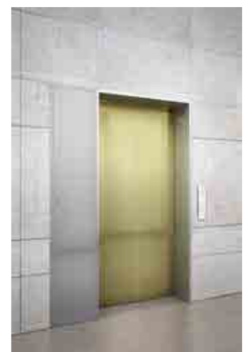
Entrance with control panel
