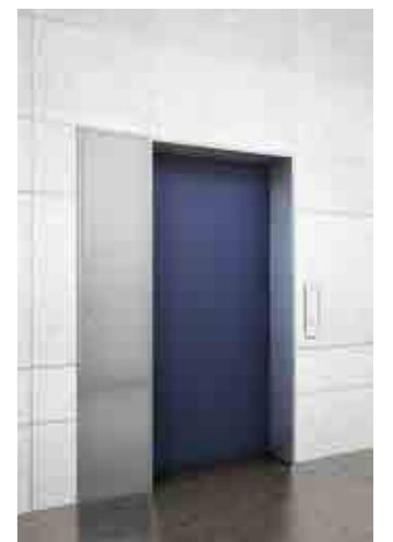
Entrance with control panel
