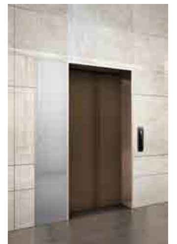
Entrance with control panel
